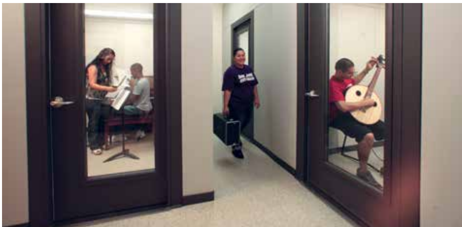
Wenger Sound-Isolation Rooms used as Music Practice Space - San Jose City College, San Jose, California
