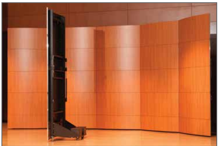
Use tool to raise top panel to its full height.
