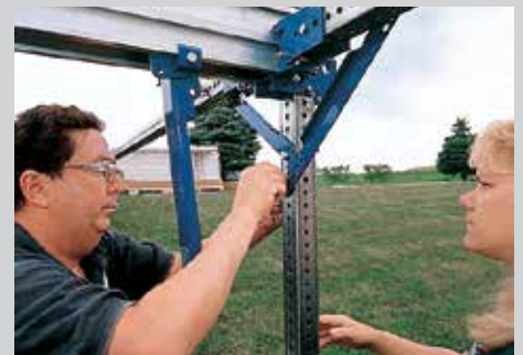
STRATA has self storing diagonal bracing that provides lateral stability and does not require any tools. STRATA'S diagonal bracing is all you need for floors up to 4' (122 cm) high.
