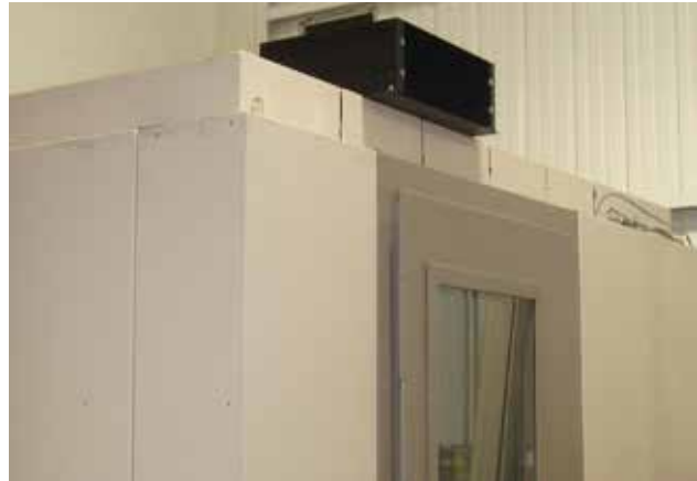
Black Box mounted to top of Ceiling Panels (Preferred Position)
