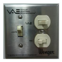
The ventilation fans draw air out of the room and replace it with ambient air from outside the room. Using this switch, it is recommended that the fans be turned on anytime the room is occupied. Fan operation can be verified by looking for airflow by holding a lightweight piece of paper (or similar material that will react to the flow of air) near the ventilation registers.
