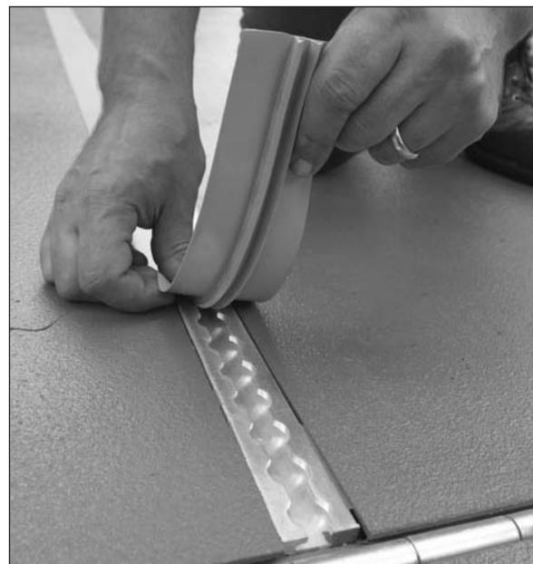
12. Press a fill strip into each channel in the stage floor. Make certain a strip is fully inserted into each channel to prevent edges and gaps which can trip performers or snag equipment.
