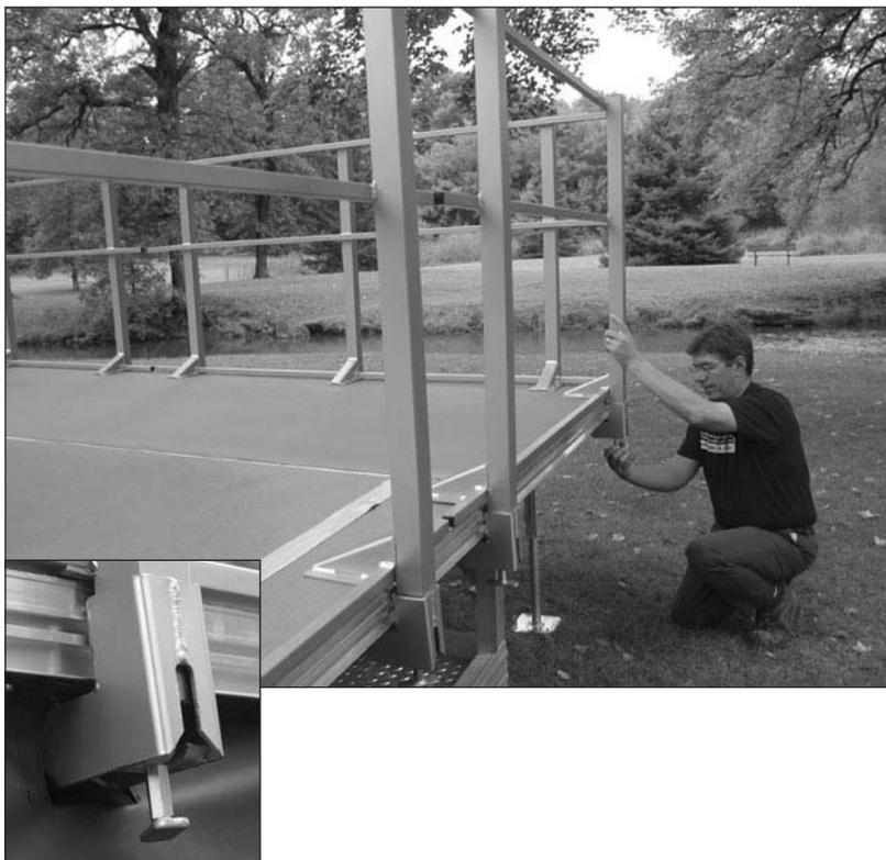
2. After the feet of the railing section are fully inserted over the edge of the stage, lift each lower foot until you can slide the T-handle to the bottom of the foot, then tighten the T-handle to clamp the foot securely (see inset photo). Once all railing sections are attached, check to make certain each section is firmly secured.
