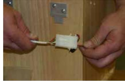
6. Connect the four cables to the loudspeakers using their mating, 4-terminal connectors.
