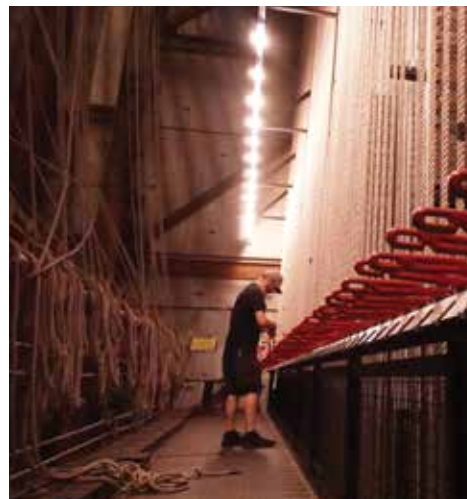
Gallery rope locks are shown here in the open position during stage level operation.
